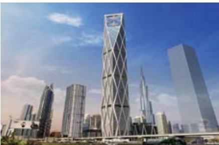
Project : SRG TOWER MEP Consultant : Erga Progress Engineering Consultants MEP Contractor : International Electro-Mechanical Services Co. LLC Location : Dubai, UAE Year : 2024
