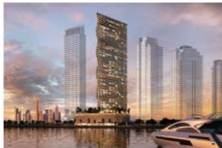
Project : Mar Casa MEP Consultant : Prasoon Design Studio FZ-LLC MEP Contractor : Al Arabia Electro Mechanical LLC Location : Dubai Maritime City, Dubai, UAE Year : 2024
