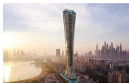
Project : Como Residences MEP Consultant : Group Consult International MEP Contractor : Al Futtaim Engineering Location : Palm Jumeirah, Dubai, UAE Year : 2025
