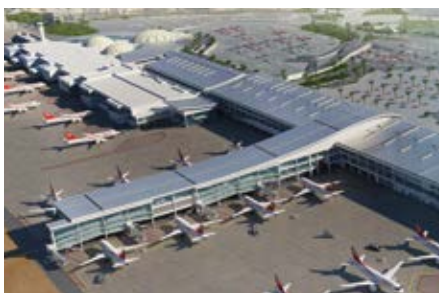
Project : New Passenger Terminal Building MEP Consultant : Parsons MEP Contractor : Binladin Contracting Group LLC Location : Sharjah Airport, UAE Year : 2024
