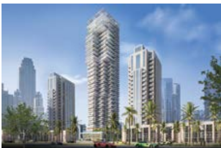
Project : Fairmont Residences Solara Tower MEP Consultant : Group Consult International MEP Contractor : Bhatia Power Electromechanical Location : Dubai, UAE Year : 2025
