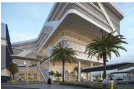
Project : DP World Head Office MEP Consultant : Design & Architecture Bureau (DAR) MEP Contractor : Al Ghurair MEP LLC Location : Dubai, UAE Year : 2025
