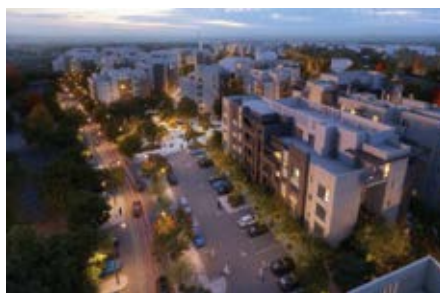
Project : 493 housing units 29 residential buildings Sidra neighborhood MEP Consultant : HAJ Gulf Consultancy / AJ Consult MEP Contractor : HOMES Contracting Company Location : KSA Year : 2025
