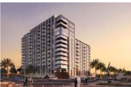
Project : Manarat Living Phase-2 MEP Consultant : Ultra Architecture consultancy (U+A) MEP Contractor : Power spray Electromechanical Sole Proprietorship LLC Location : Abu Dhabi, UAE Year : 2024
