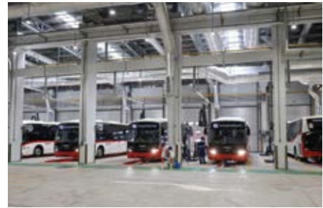
Project : RTA Bus Depots MEP Consultant : Al Turath Engineering Consultants MEP Contractor : Bin Hanif Electromechanical LLC Location : Dubai, UAE Year : 2024
