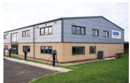
Project : LEW Head Office Contractor : Analogue Electrics Location : Lincolnshire, England Year : 2025
