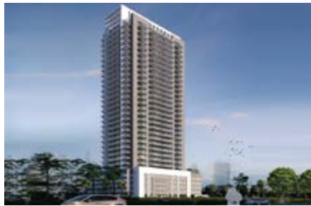
Project : The Violet Tower in JVC MEP Consultant : CONIN International Consultants MEP Contractor : Al Ghurair MEP LLC Location : Dubai, UAE Year : 2024
