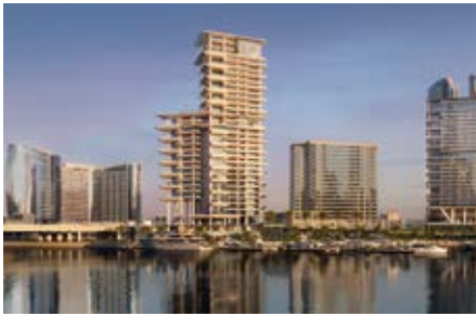
Project : Vela by Omniyat MEP Consultant : Rice Perry Ellis MEP Contractor : Menasco Mechanical Contracting Co. LLC Location : Business Bay, Dubai, UAE Year : 2024
