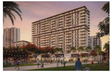
Project : Town Square Nshama MEP Consultant : Symphony Engineering Consultants L.L.C MEP Contractor : Gincio Electrical & Sanitary Contracting Co.L.L.C Location : Dubai, UAE Year : 2024
