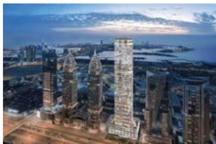
Project : Iconic Tower MEP Consultant : SEED Engineering Consultants MEP Contractor : EMT Electromechanical Works L.L.C Location : Dubai Internet City, Dubai, UAE Year : 2025
