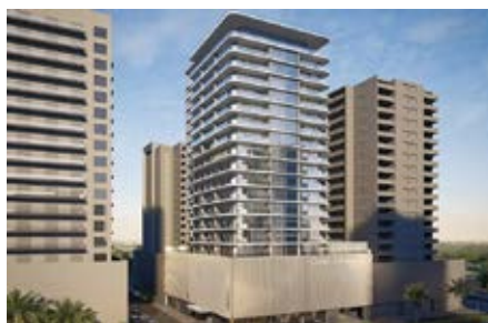
Project : Livel Residenza- JVC MEP Consultant : Archcorp Architectural Engineering MEP Contractor : Al Amal Electromechanical L.L.C. Location : Dubai, UAE Year : 2024
