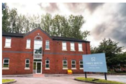
Project : Abbey House Dental Surgery Contractor : Penkhull Electrical Location : Stoke on Trent, England Year : 2024
