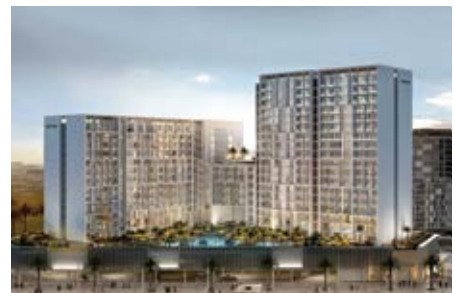
Project : Jannat Midtown MEP Consultant : Jouzy Consulting Engineers MEP Contractor : EMAC Electromechanical LLC Location : Dubai, UAE Year : 2024
