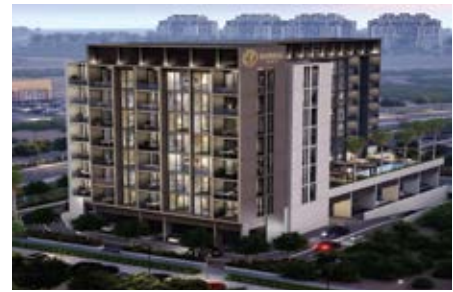
Project : Imperial Residence MEP Consultant : MAKES Engineering Consultancies MEP Contractor : Al Sarya Technical Artistic Location : Production City, Dubai, UAE Year : 2024
