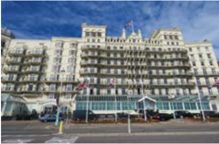
Project : Brighton Grand Contractor : Airtemp Location : Brighton, England Year : 2018
