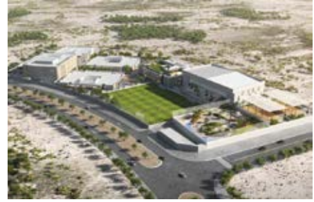
Project : Dubai English Speaking School MEP Consultant : Graphite International MEP Contractor : Al Shirawi Electrical & Mechanical Company Location : Academic City, Dubai, UAE Year : 2024
