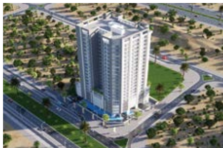
Project : Time 3 Residential Building MEP Consultant : HADI Consulting Engineering MEP Contractor : Bayan Construction LLC Location : Dubai, UAE Year : 2025
