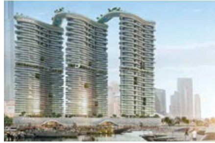
Project : Damac Bay 1 by Cavalli MEP Consultant : KEO Engineering Consultant MEP Contractor : Menasco Electromechanical Location : Damac Bay, Dubai, UAE Year : 2024
