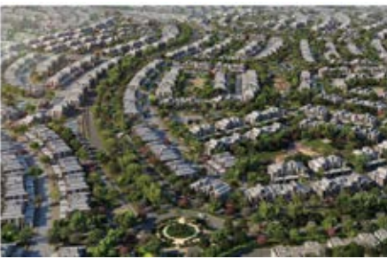
Project : Muuddoonn Central Park Phase 7&8 MEP Consultant : Dubai Holding Real Estate MEP Contractor : GESCO Star Electrical & Sanitary Contracting Location : Dubai, UAE Year : 2024
