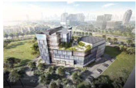
Project : Asan Gastroenterology Specialty Hospital MEP Consultant : HDP Overseas Ltd MEP Contractor : Pluto Electromechanical Cont. LLC Location : Dubai, UAE Year : 2024
