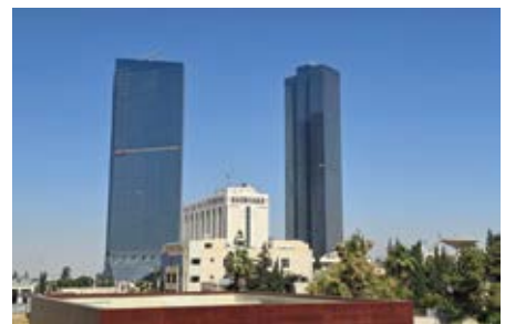
Project : Jordan Gate, North Tower MEP Consultant : Al Nasser + Partners Architect & Engineers MEP Contractor : Jet Contracting Location : Jordan Year : 2024
