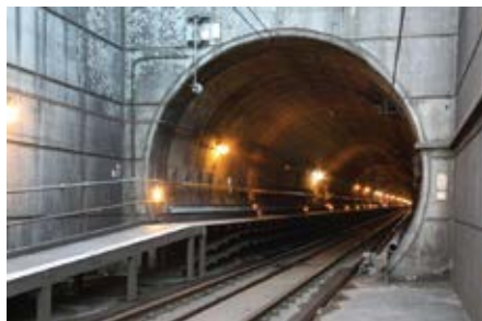
Project : Stansted Tunnel Contractor : J Murphy & Sons Location : Stansted, England Year : 2022
