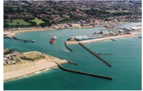
Project : Shoreham Harbour – GRP Tray Contractor : DW Electrical Location : Shoreham, England Year : 2020
