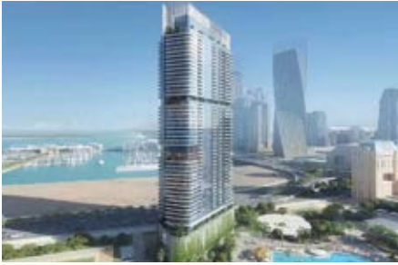
Project : Habtoor Grand Residences MEP Consultant : John R Horris MEP Contractor : China Railway 18th Bureau Group LLC Location : Dubai, UAE Year : 2024
