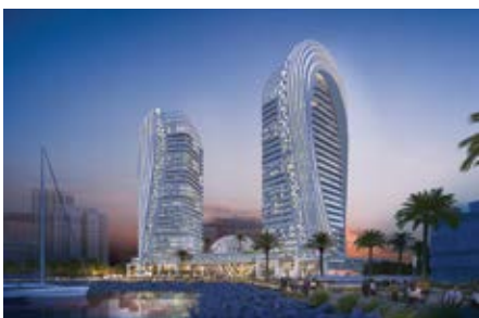
Project : Azure Twin Tower MEP Consultant : FD Consult MEP Contractor : MechaTronics WLL Location : Lusail, Qatar Year : 2024
