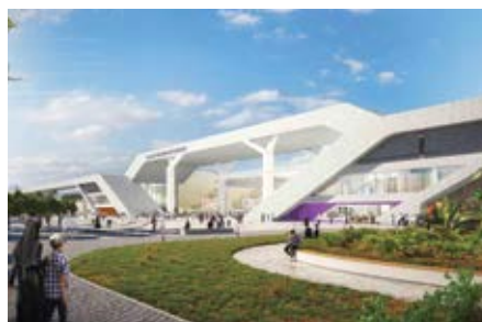
Project : DEC Campus Legacy MEP Consultant : Egis Engineering Consultant MEP Contractor : Al Futtain Engineering Location : Dubai Exhibition Centre, Dubai, UAE Year : 2024
